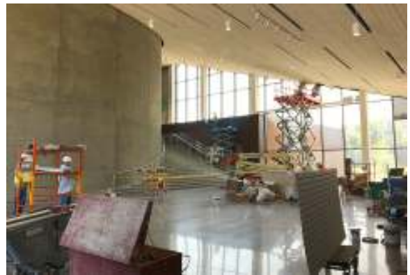
Front entrance of the Bell currently under construction.
