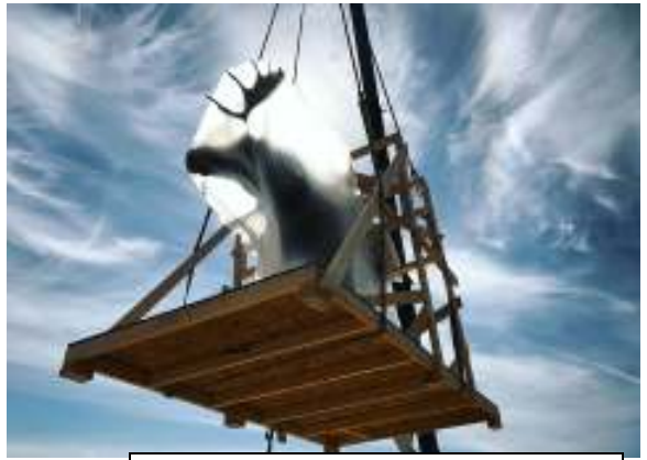
A taxidermied moose is hoisted off a truck at the new museum location.
